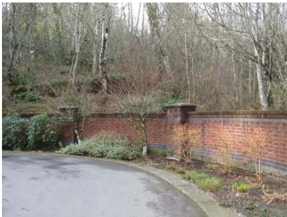
Main Gate Brick Wall and Concrete Cap
