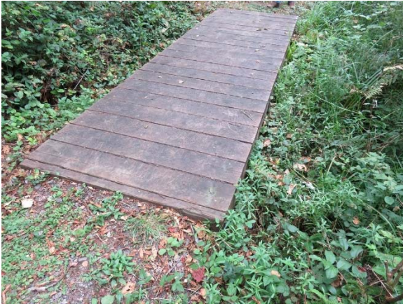
One of Three Trail Bridges
