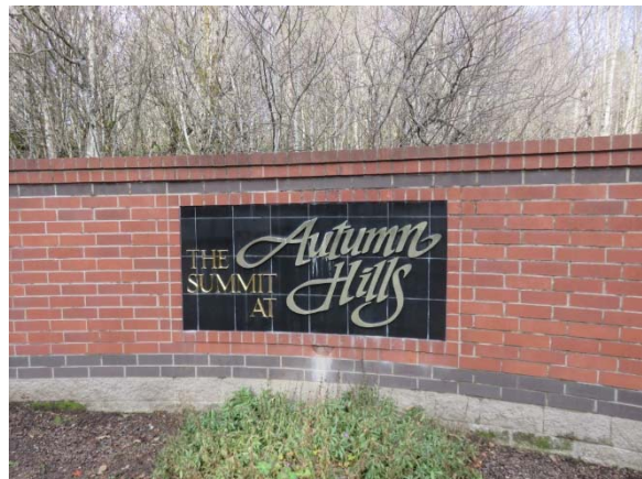
Main Gate Brick Wall and Concrete Cap
