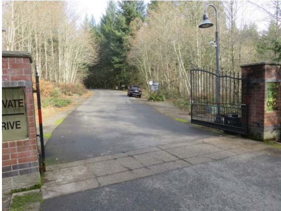
Both Swinging Gates at Main Gate
