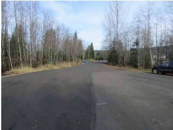
Newly Patched Area of Asphalt
