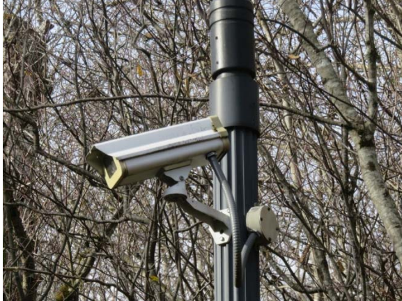
Surveillance Camera at Main Gate
